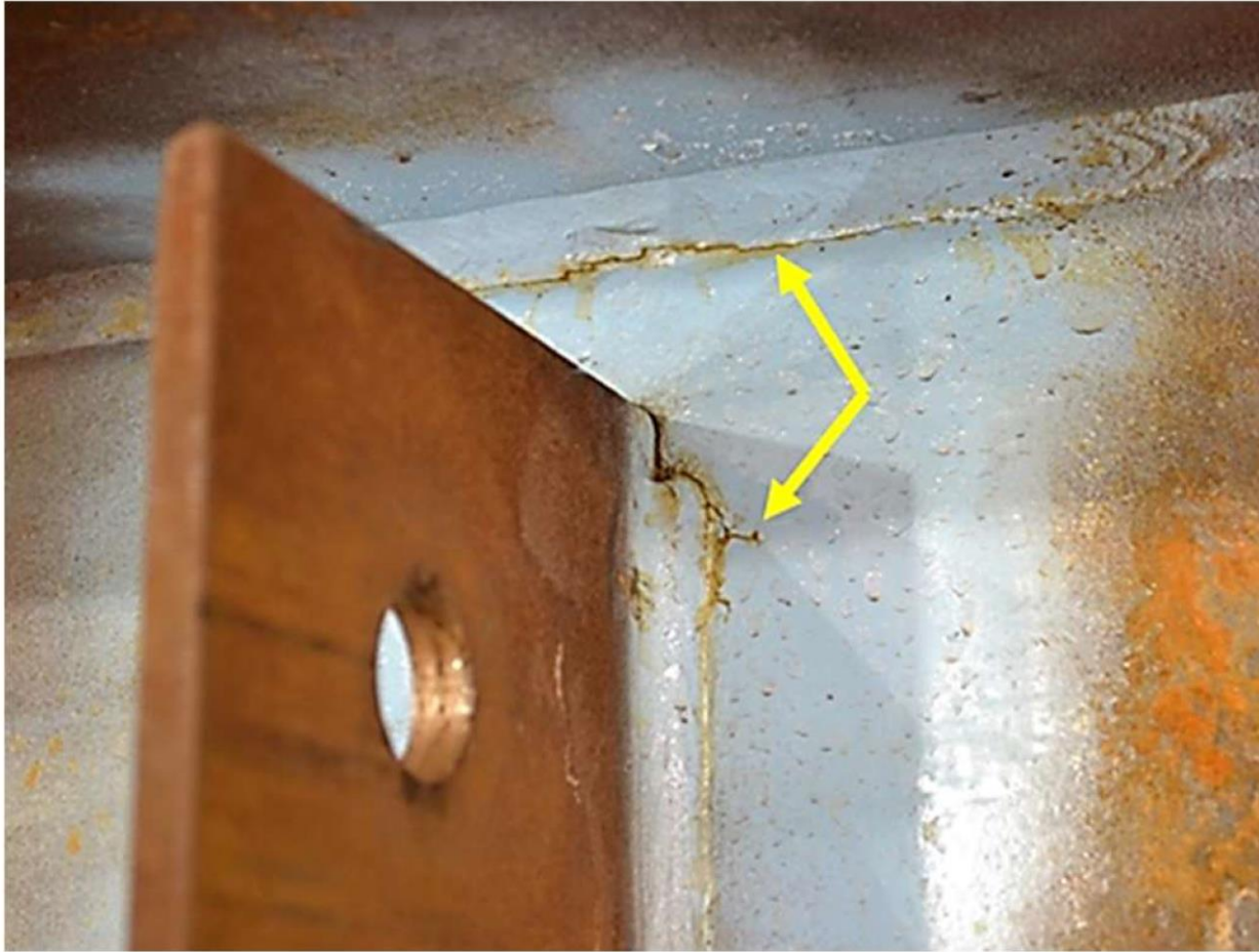
Distortion Induced Cracking
